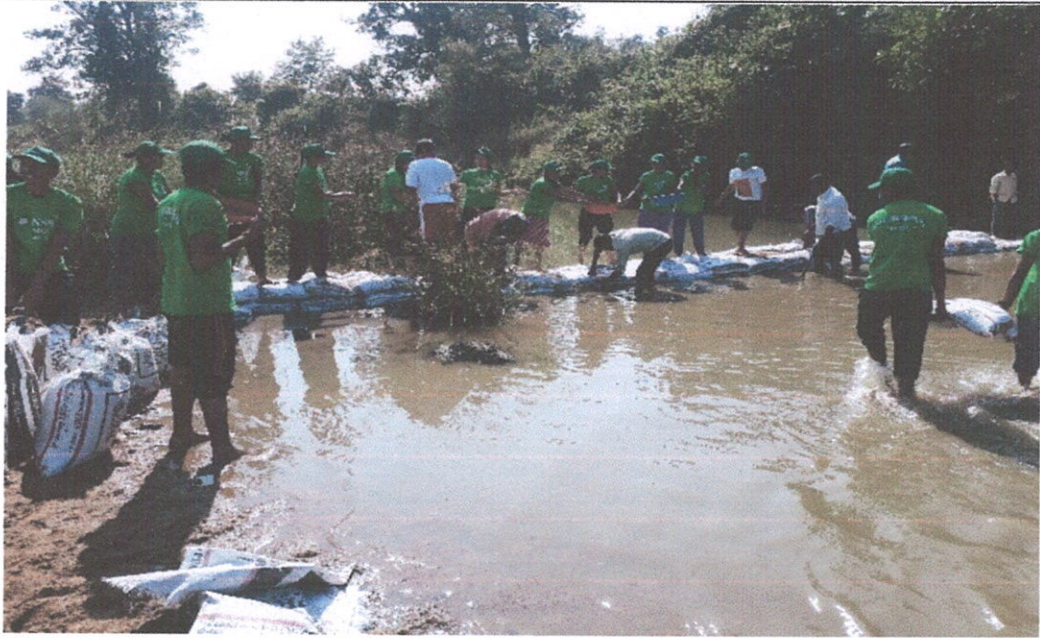
Construction of Kuchha Dam by students
